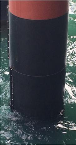
RETROWRAP STD2 is a wraparound corrosion protection solution for inshore splash zone and underwater corrosion protection for piles, pipelines and risers. STD2 is specifically designed to endure the rough conditions through the splash zone at semihard wave conditions and moderate temperature variations.
